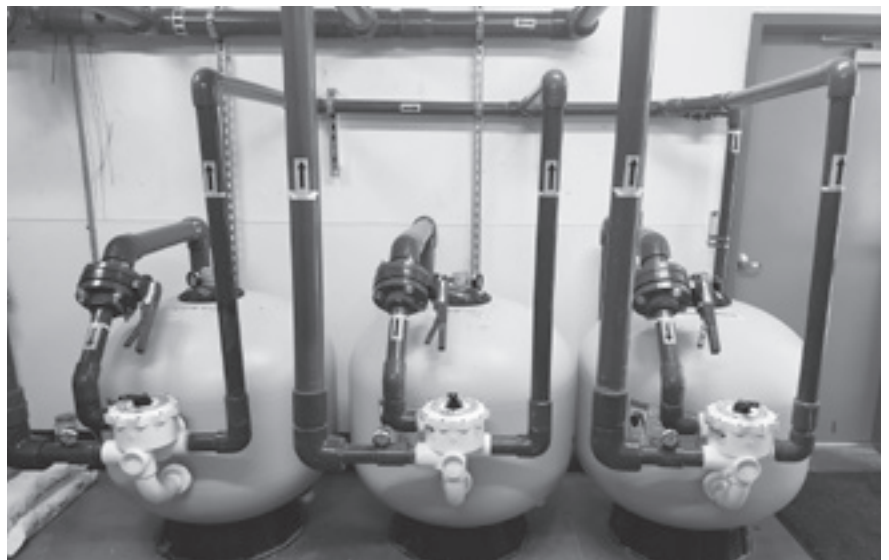
Commercial Pool system with Colonial BFVs
