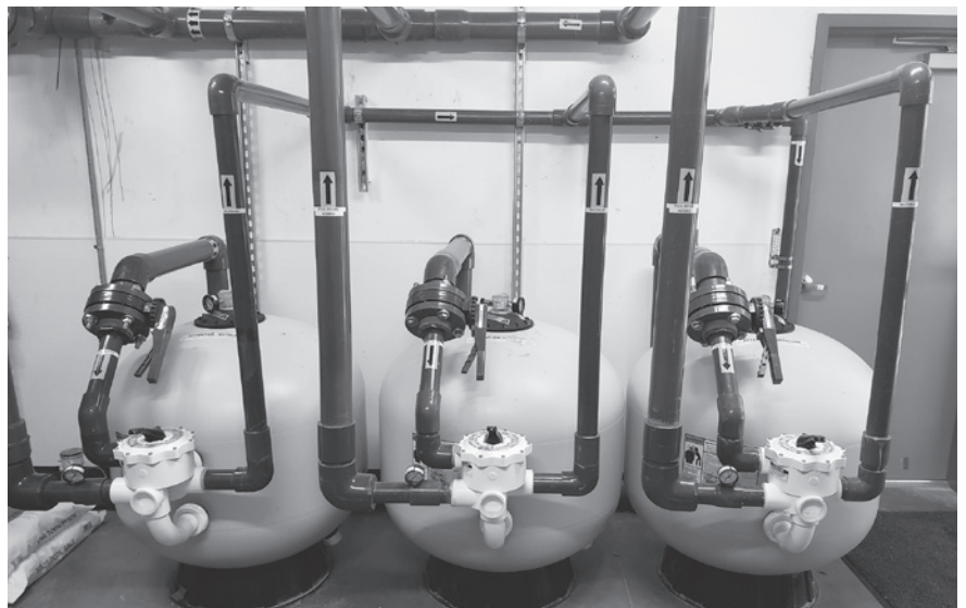
Commercial Pool system with Colonial BFVs
