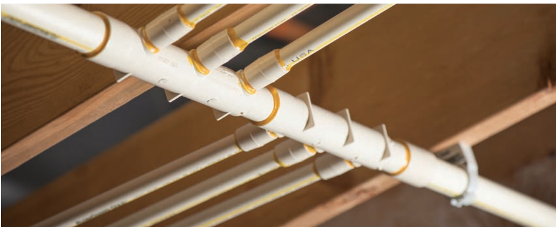
Proper support for a horizontal installation.
