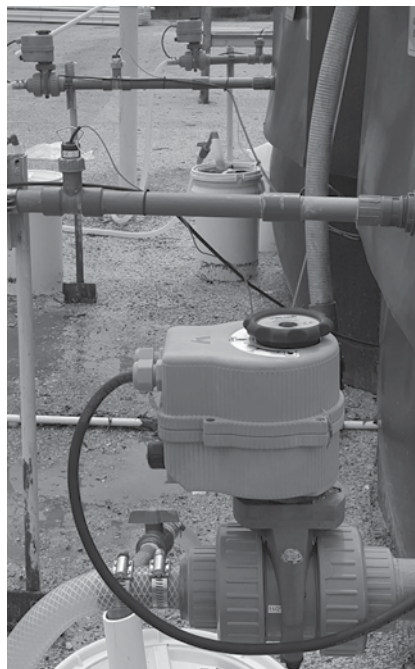
Industrial TUBV with Electric Actuators on a chlorine dispensing system in Florida.
