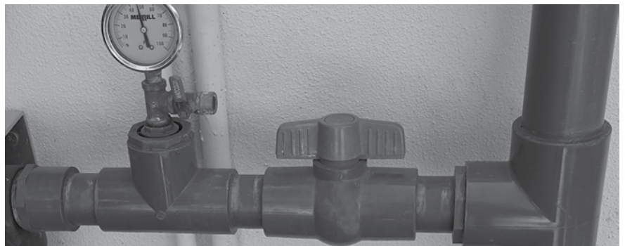
2" Compact Valve on Water Treatment system in St. Thomas USVI.
